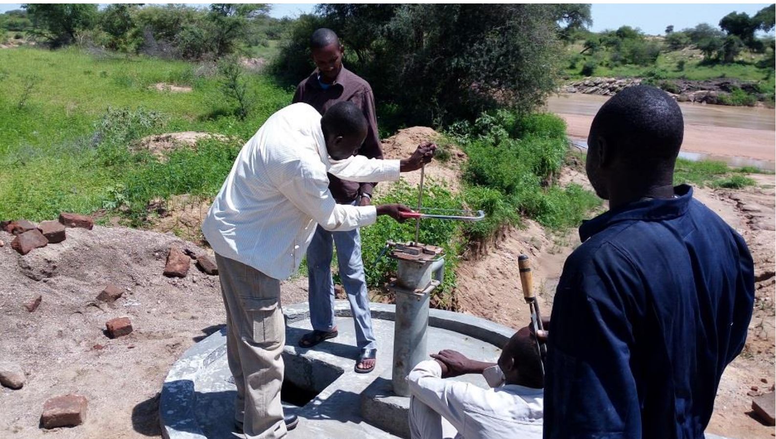
Figure 7: Completed sub-surface dam and water pump for Makada village
