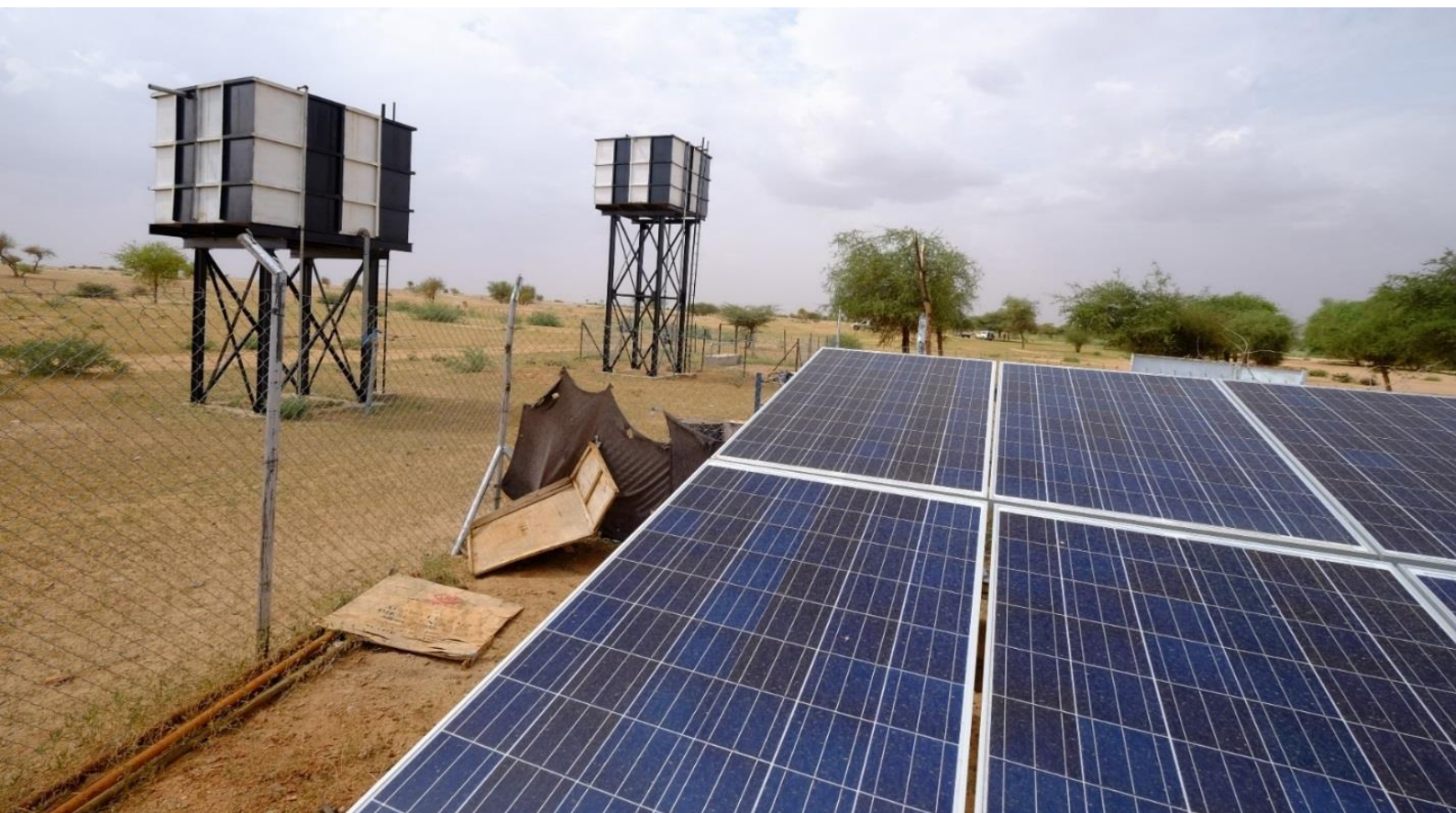
Figure 6: Solar water supply system- Garajeem village, Korno locality, North Darfur
