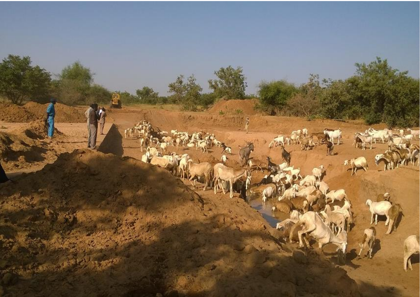
Figure 2: Sub-surface dam in Furro, West Darfur is in progress
